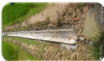
Rectification of irrigation cum drainage channel with cement slabs
